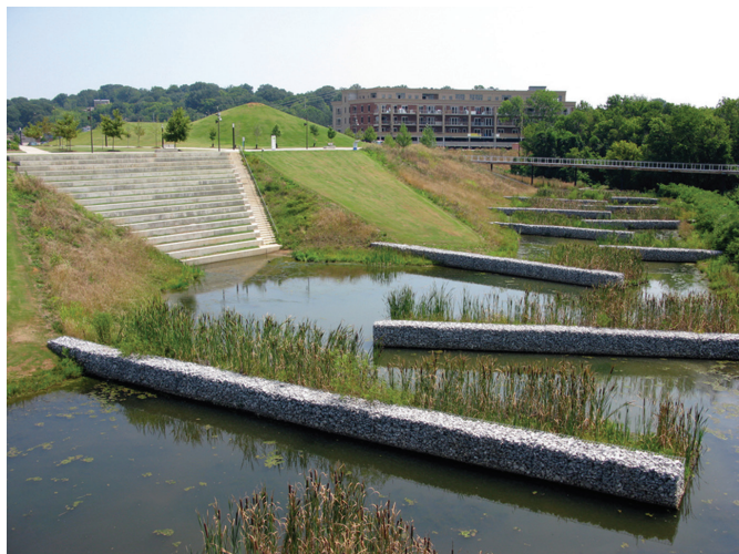
A constructed wetland built in a community park in a formerly industrialized area of Chattanooga, TN collects and cleans runoff before it flows into the Tennessee River
