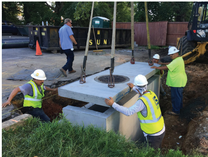
Local workers install stormwater management device in Prince George's County, MD
