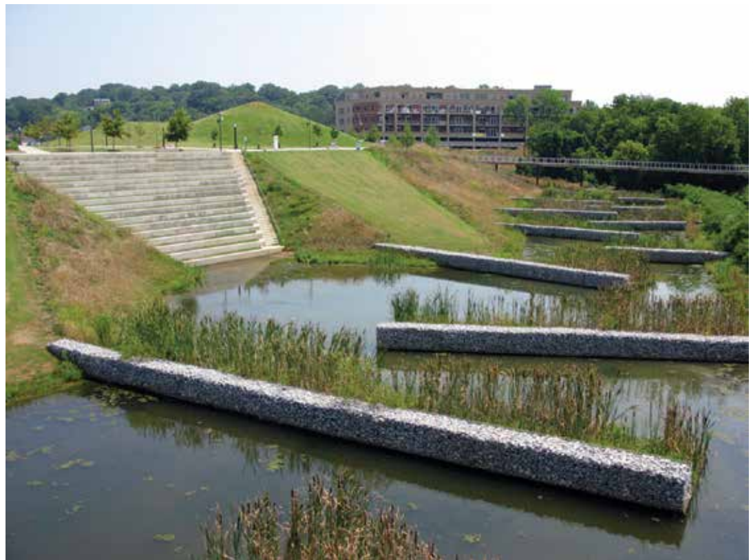
A constructed wetland built in a community park in a formerly industrialized area of Chattanooga, TN collects and cleans runoff before it flows into the Tennessee River.
