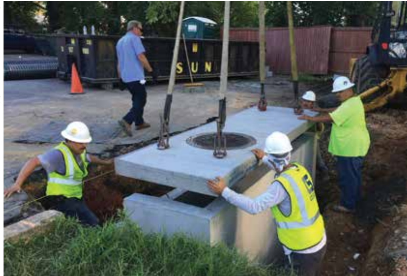
Local workers install stormwater management device in Prince George's County, MD
