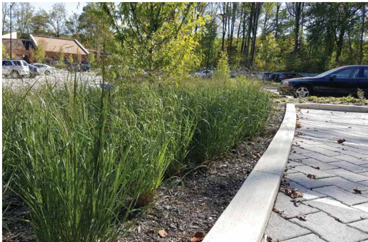
Permeable pavers in the Brookside Gardens parking lot in Wheaton, MD
