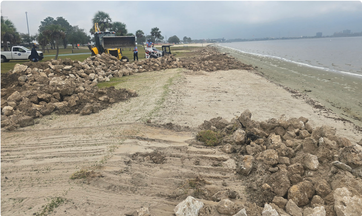
Crews install rock barriers to help mitigate beach erosion. Photos courtesy of Lake Charles.
